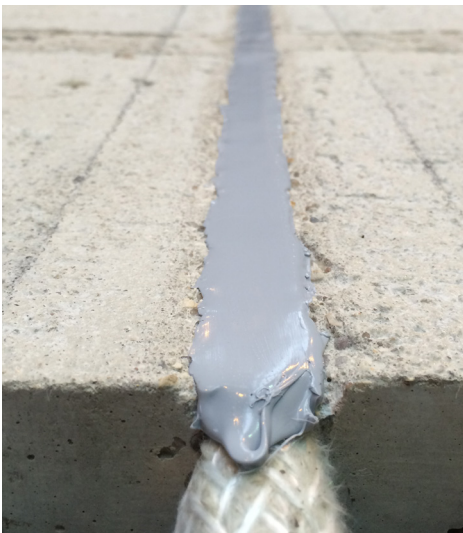
FJ203 bonded with FO142/3 Intutac + FS703 Intusil for waterproofing: EI240
